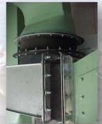
Style 600 Rubber Flue Duct Expansion Joints and Navy Fan
